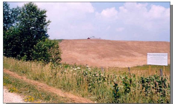
Land is ready for seeding
