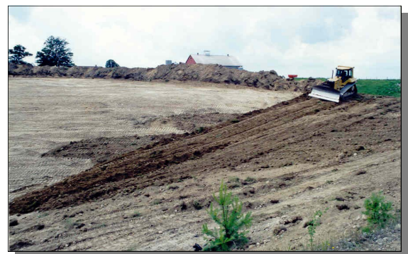
Spreading topsoil on a newly graded pit face
